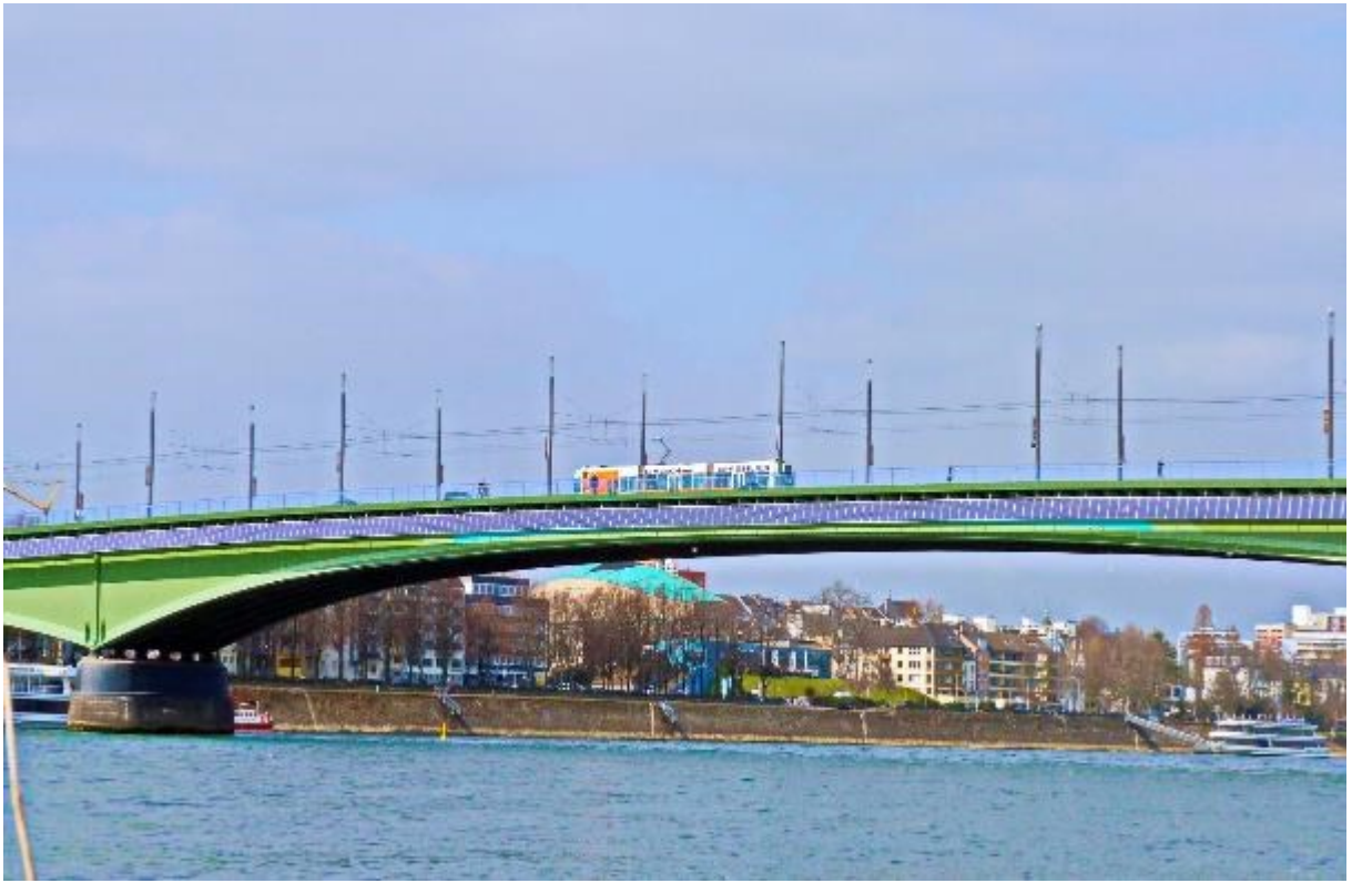
Solar-Brücke in Bonn (Kennedy-Brücke)
